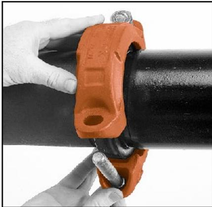
**4 HOUSINGS—** Place the coupling housing halves over the gasket making sure the housing keys engage the grooves. Insert bolts and turn nuts finger tight.
