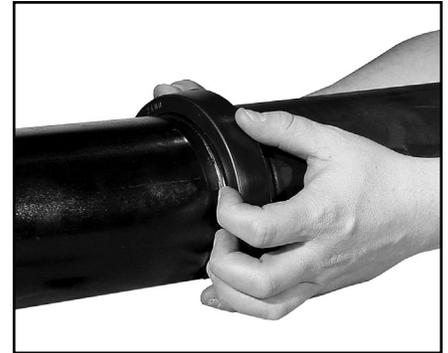
**3 ALIGNMENT—** After aligning the two pipe ends, pull the gasket into position centering it between the grooves on each pipe. On couplings 10" and larger, flip or roll the gasket into centered position.
