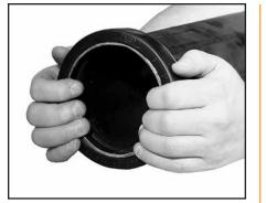
**2**GASKET INSTALLATION— Slip the gasket over the pipe end, making sure the gasket lip does not overhang the pipe end.
