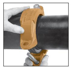
**HOUSINGS**— With one nut unthreaded to the end of the bolt, unthread the other nut completely and swing the coupling housing halves over the gasket, making sure the housing keys engage the grooves. Insert the bolt and turn the nuts finger tight.
