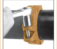
**5** TIGHTEN NUTS— Tighten the nuts alternately and equally to the specified bolt torque. The housing bolt pads must make metal-to-metal contact.
